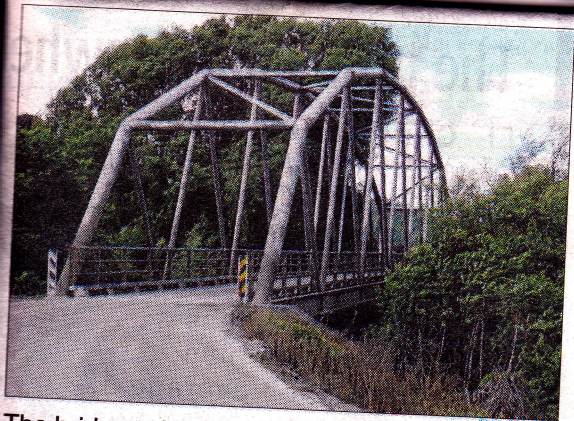
The bridge at Wilsons Rd, Parakao.
